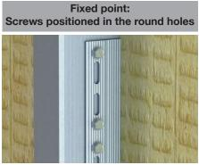
• Fixed point: The screws must be positioned in the round holes to avoid vertical movement.
