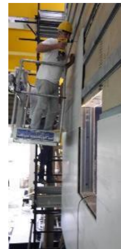
Exterior wall panels fixing
