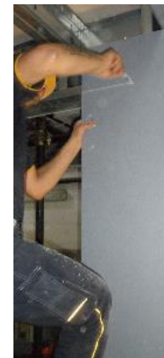
Interior wall panels fixing
