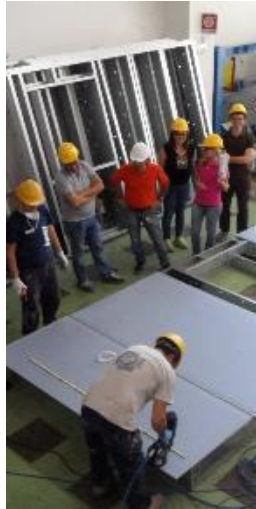
Exterior wall panels nailing
