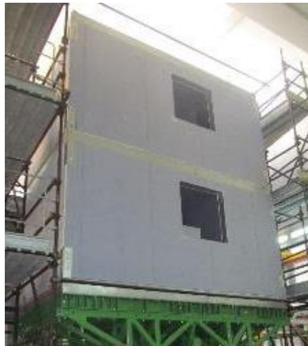
Whole bare structure
