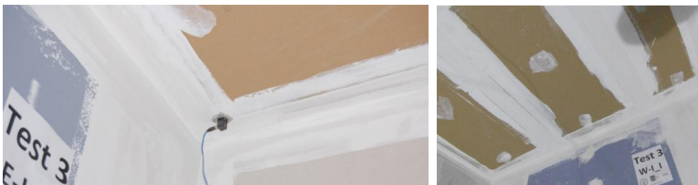
Very low damage observed for suspended ceiling
