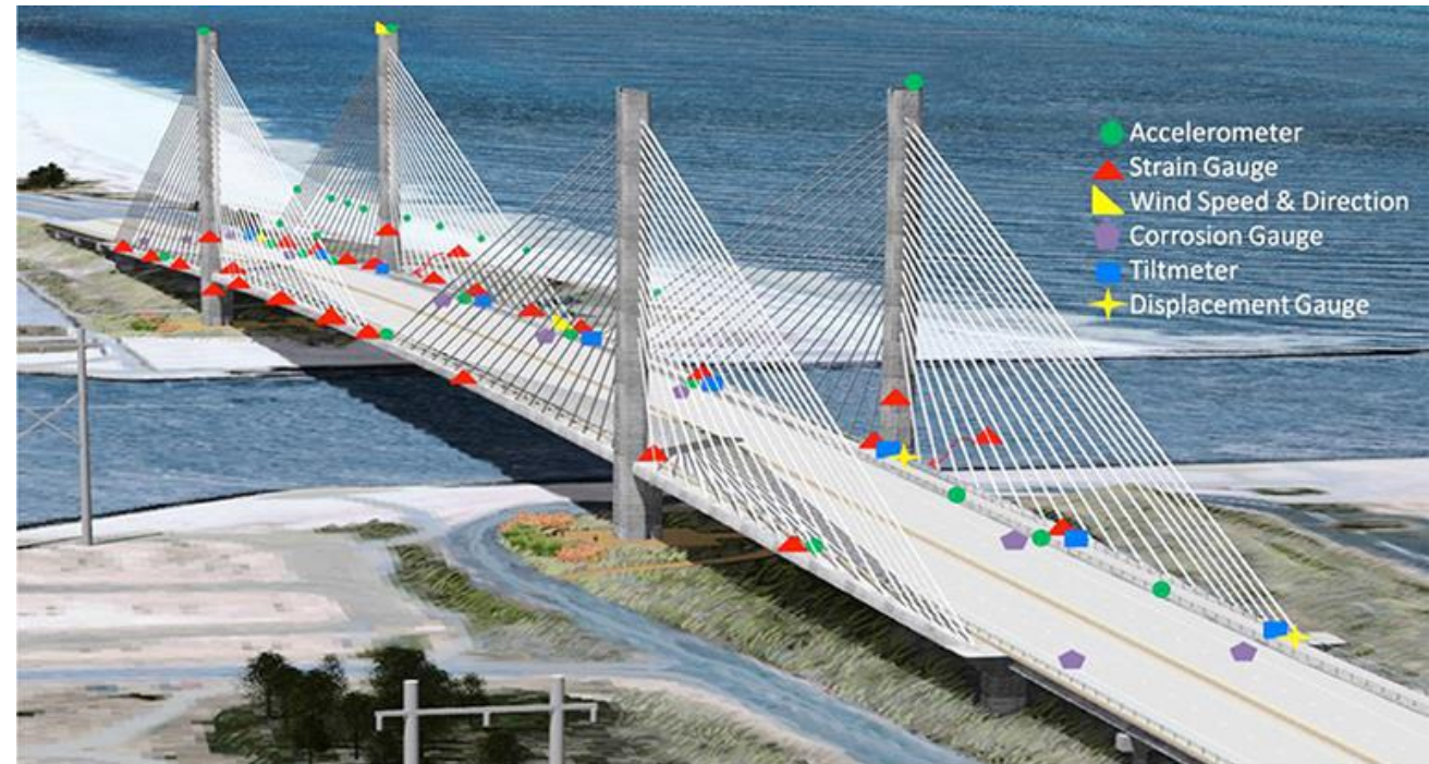
Al-Khateeb et al. «Structural Health Monitoring of a Cable-Stayed Bridge Using Regularly Conducted Diagnostic Load Tests»
