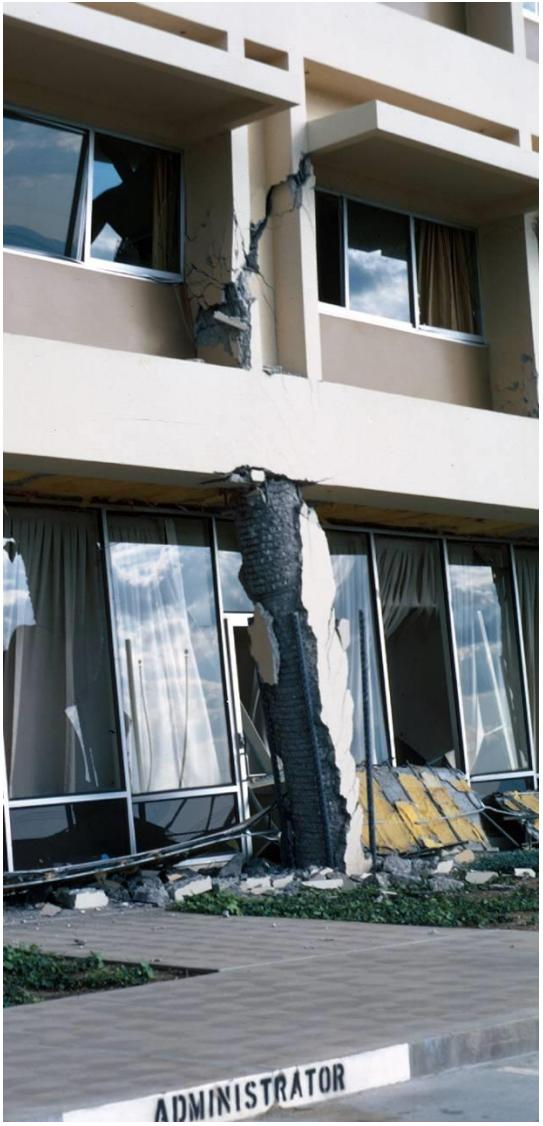
Damaged spirally-wrapped concrete pillars and shear cracks at Olive View Hospital
