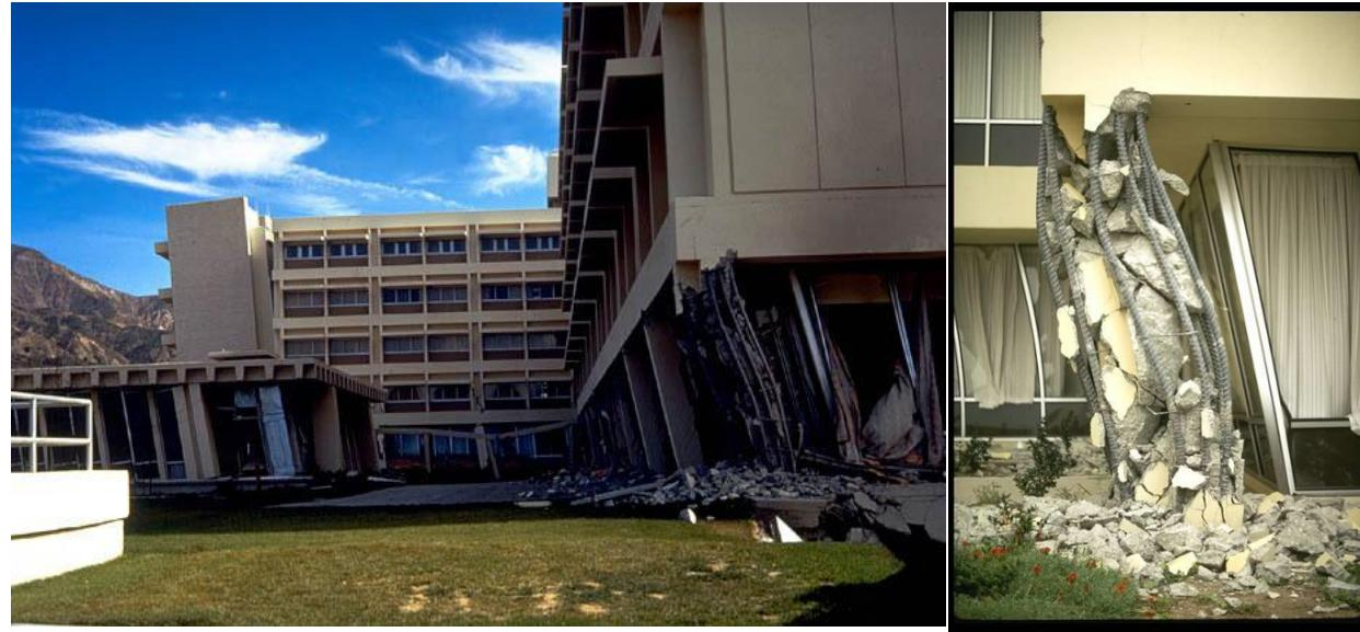
Olive View Hospital: a relative displacement with an interstory drift of 0.81 m measured at the corner columns.
