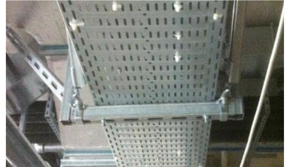
Channel frame installation
